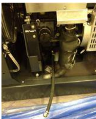
Pre-plumbed Oil Drain Line
